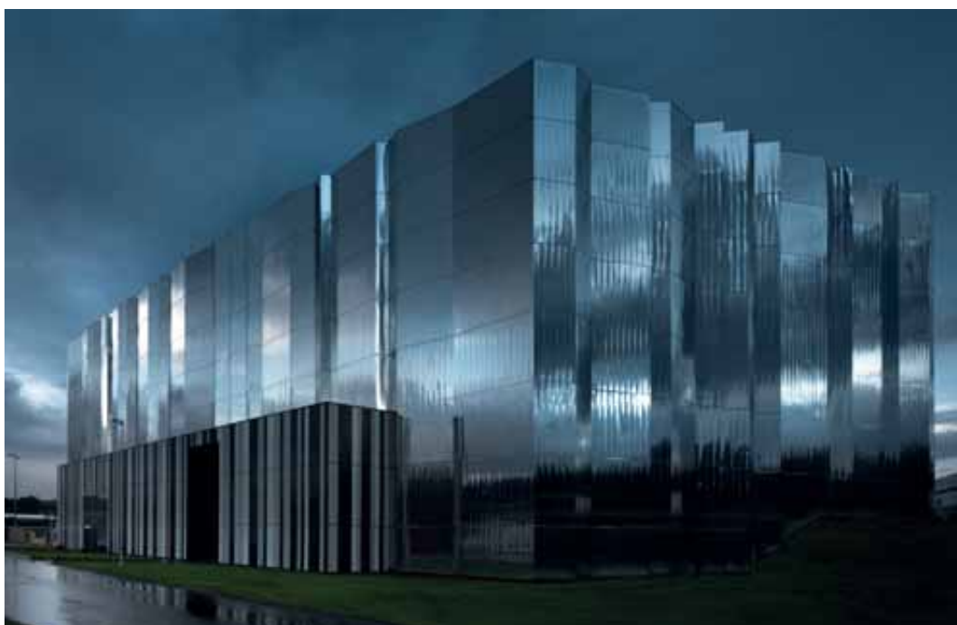
› ARTECHE new Ultra High Voltage laboratory up to 1200 kV.
