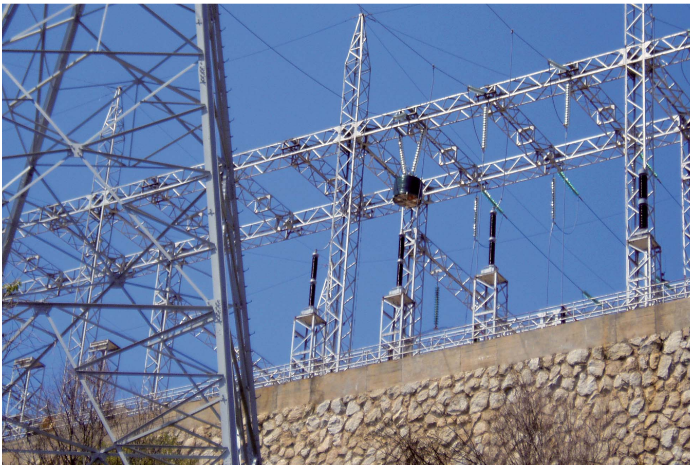
› Suspension mounted Line Traps.
