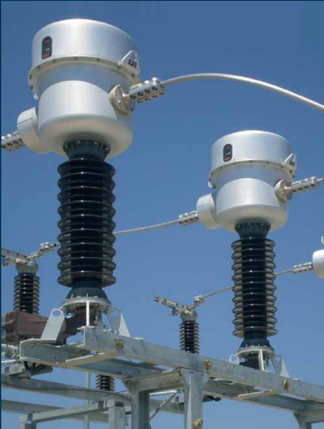
› 72.5 kV Oil-paper current transformers (CA). Endesa (Spain).
